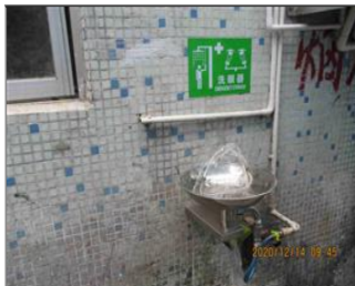
Photo first aid facilities Eyewash equipment beside spraying workshop.JPG
