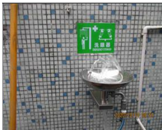
Photo first aid facilities Eyewash equipment beside chemical warehouse.JPG
